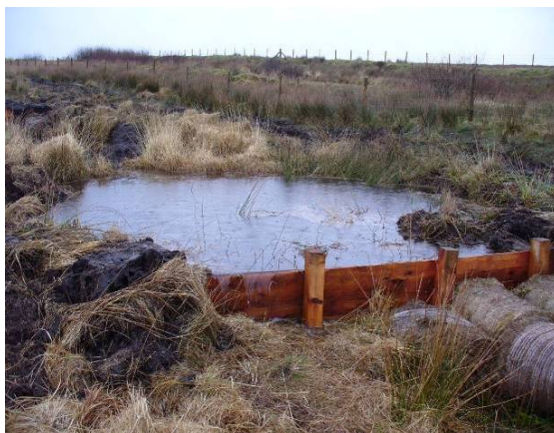
Immediately after construction of a new block
