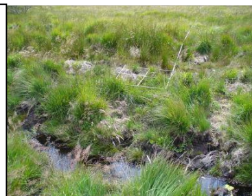
Ditch after restoration
