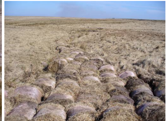
Using bales to block gullies
