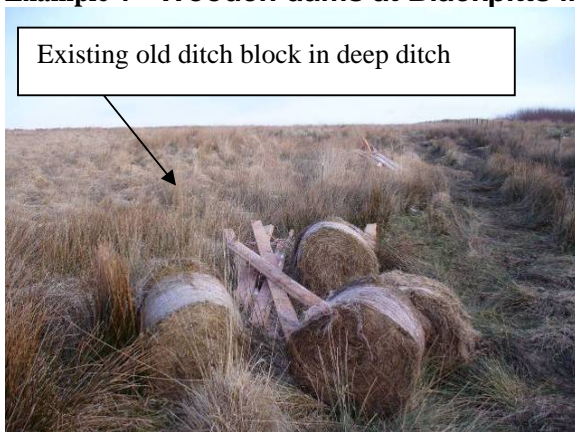
Before (construction materials at the ready)
