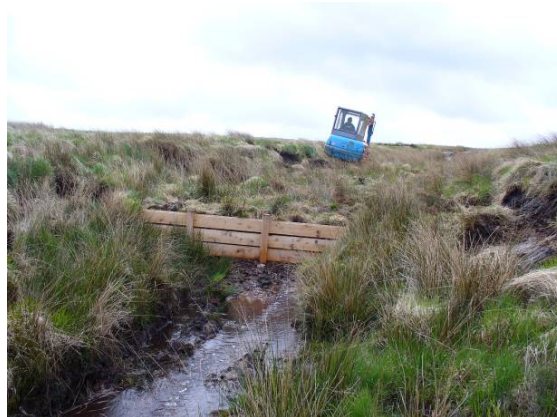
Bales being put in place
