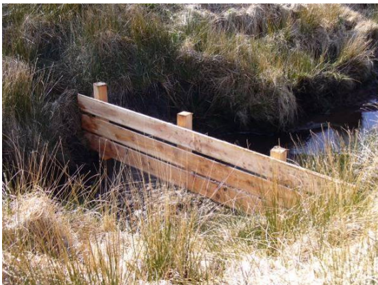
Fence across gully to hold bales
