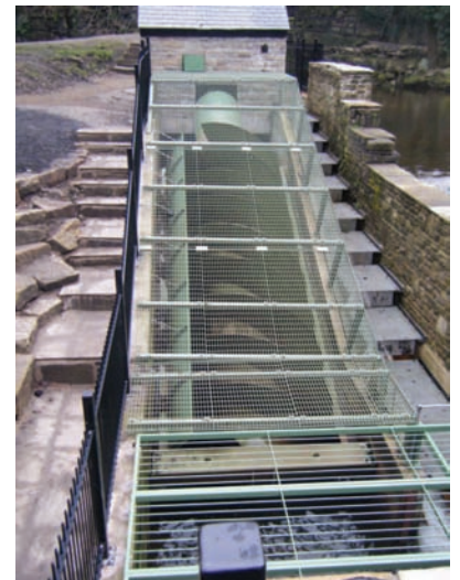
Torrs Hydro Archimedes Screw
