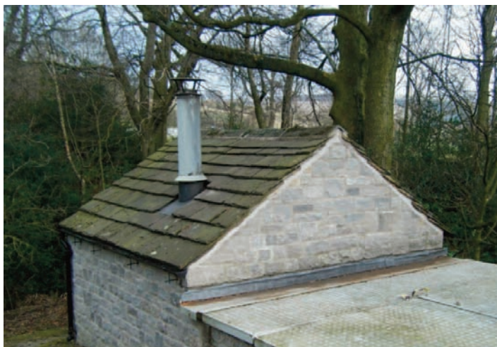
Woodchip Store and boiler house at Losehill Hall
