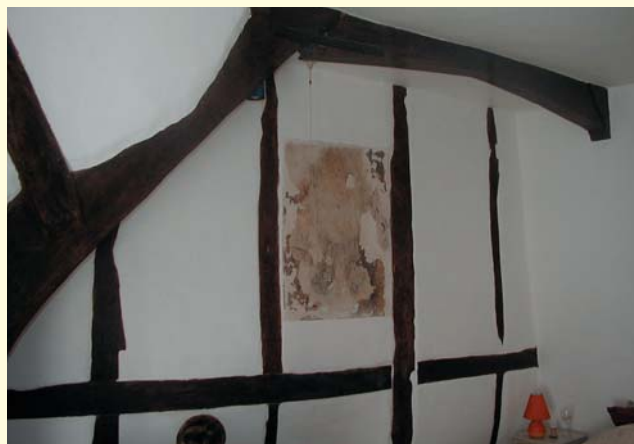
Exposed beams - Photo: Mark Clitherow
