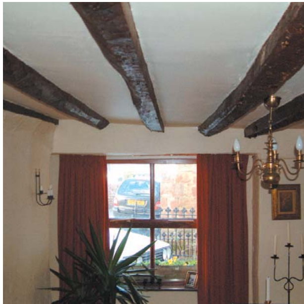
Typical exposed beams allow easy examination - Photo: Alan Simons
