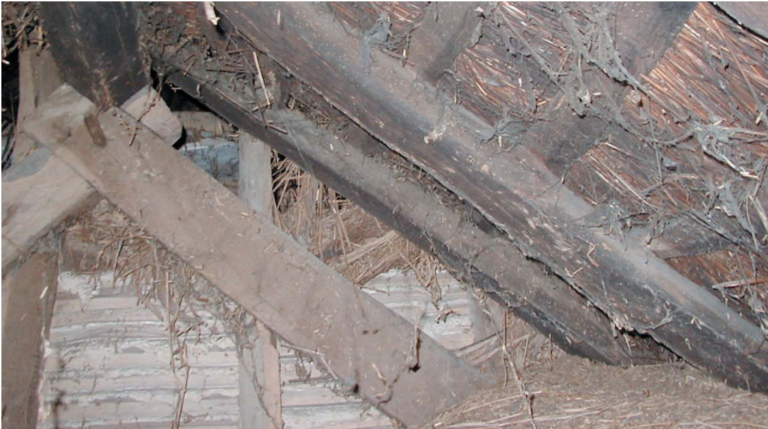
Access your roof void and inspect timbers – Photo: Mark Clitherow
