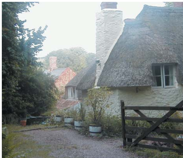
A typical thatch in good repair, the horizontal sways showing the repaired areas. – Photo: Mark Clitherow
