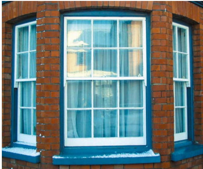
Typical sash window. Wooden windows can give good service for hundreds of years with simple maintenance. - Photo: Mark Clitherow
