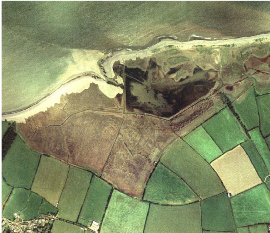
Aerial view of Porlock Shingle Ridge 2000 (post breach). The brown area shows the extent of the flooding © ENPA
