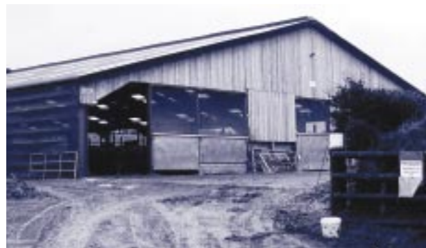
Stock Shed, Withiel Florey. A number of large developments have been approved within the National Park since the adoption of the Local Plan including large agricultural buildings. Some met with the Government's definition of major development.
