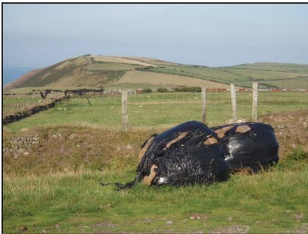
Declining condition of stone walls.
