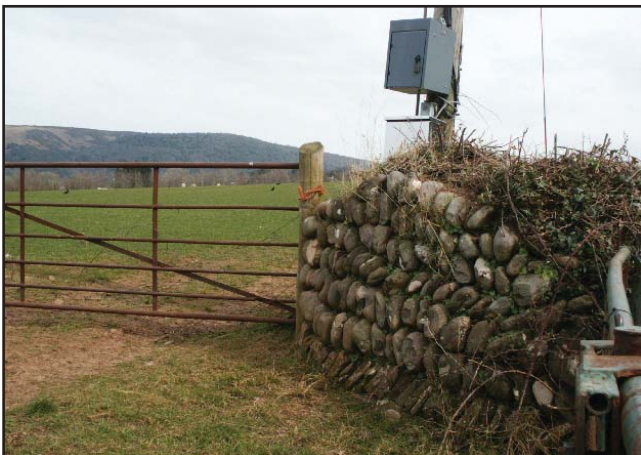
Locally distinctive hedgebanks – pebble-faced using material from the adjacent beach.
