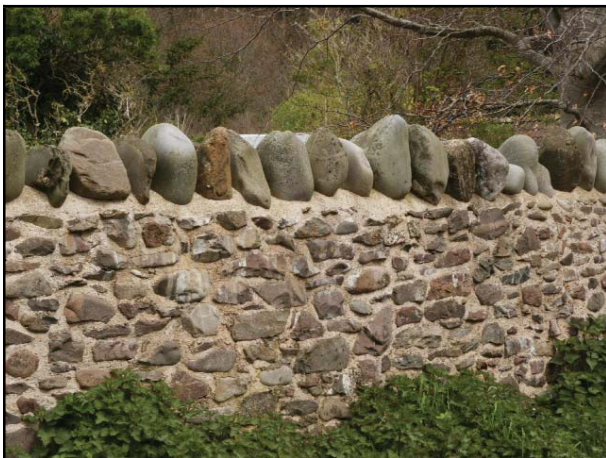
Large pebbles from Bossington beach used as a building material.
