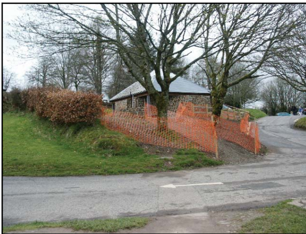
New visitor facilities at Tarr Steps
