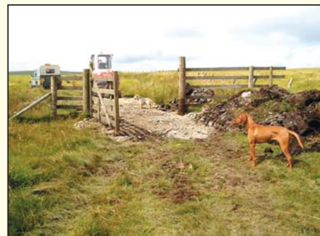
The Chains Wall permitted bridleway, before and after, where more than 100 tons of locally imported stone was used to improve the surface
