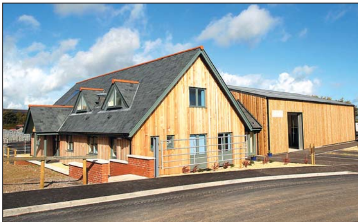
The new livestock market building which includes rainwater harvesting, air source heat pumps for the office area and solar panels for water heating funded by the Exmoor Sustainable Development Fund
