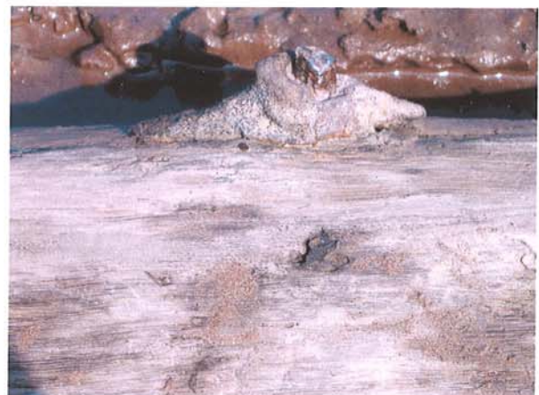
Figure 6: Nail head with ferrous concretion.
