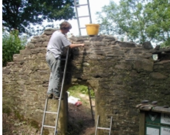
Conservation work at Burgundy Chapel, near Minehead
