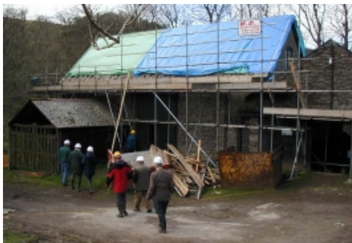
Restoration work at Simonsbath Sawmill
