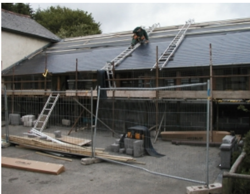
Photovoltaic roof being installed at Pinkery Education Centre
